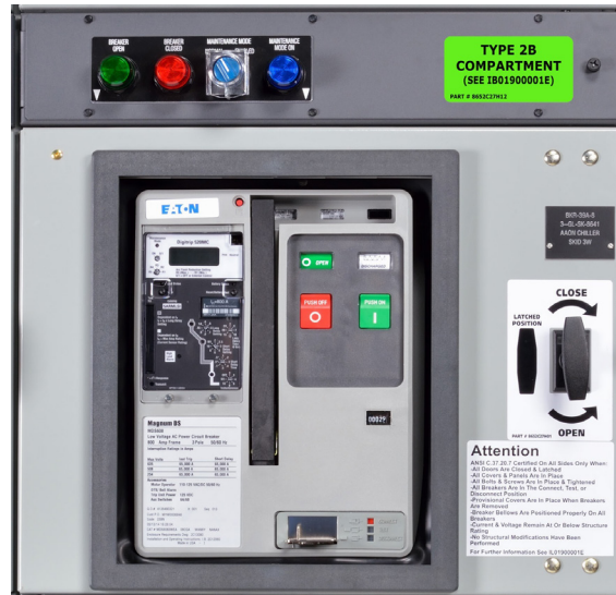
Eaton Magnum low voltage power circuit breaker with Arc flash Reduction Maintenance System to meet the arc energy reduction requirements in 240.87.
