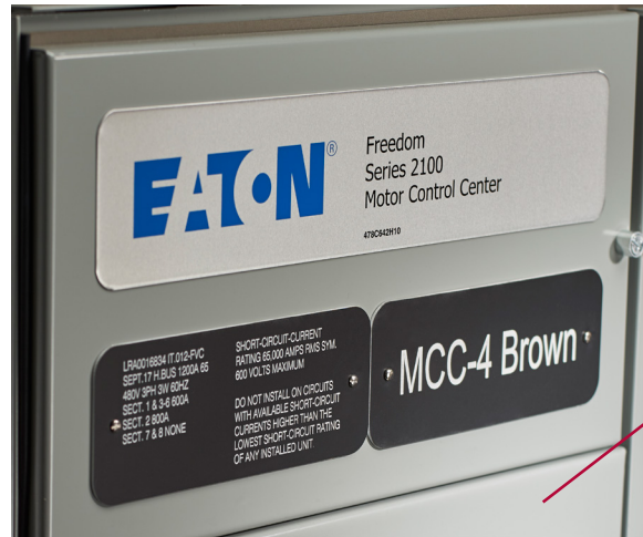
Manufacturer's nameplate with MCC SCCR marking: 65,000 A rms sym at 600V max.
